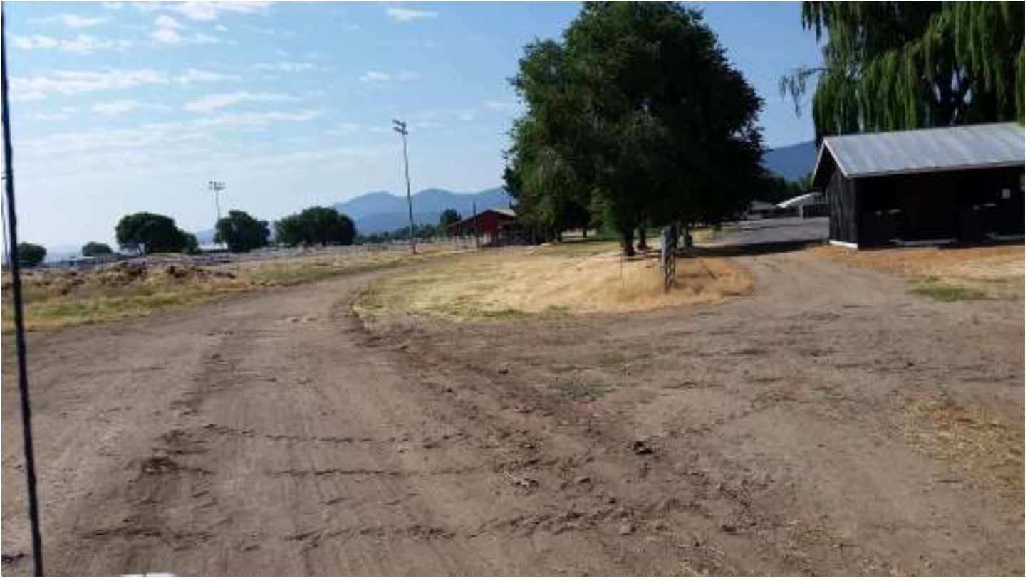
Figure 6, North Gate Roadway, portion
