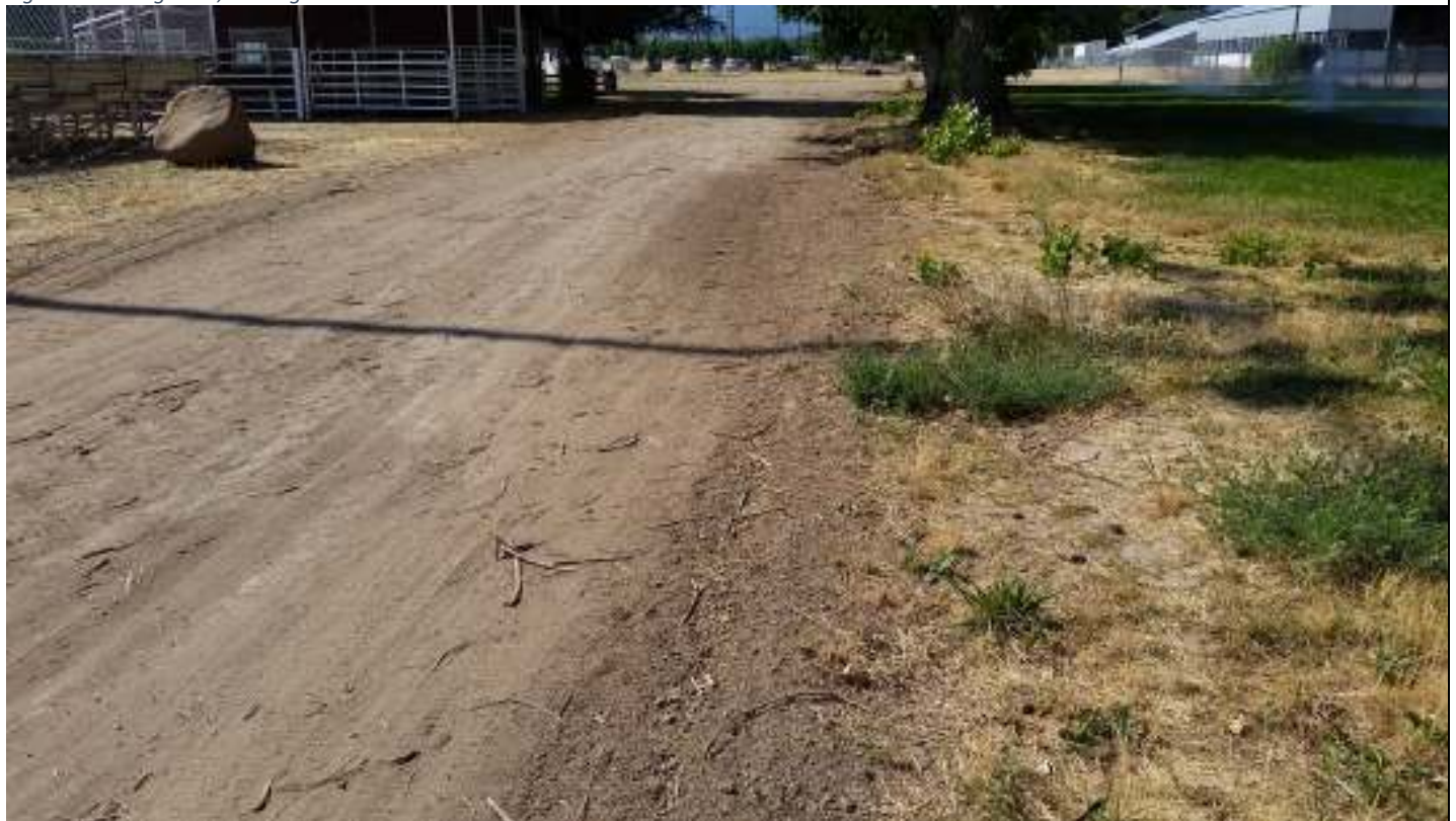
Figure 4, North Gate Roadway, portion
