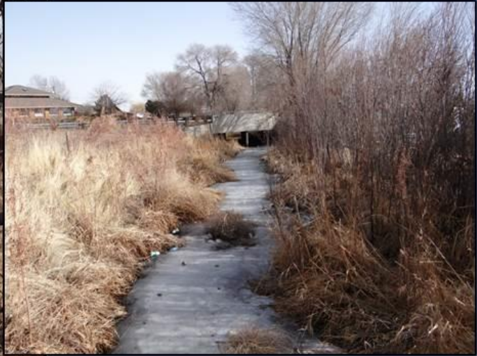
From foot bridge looking at culvert under Main St.
