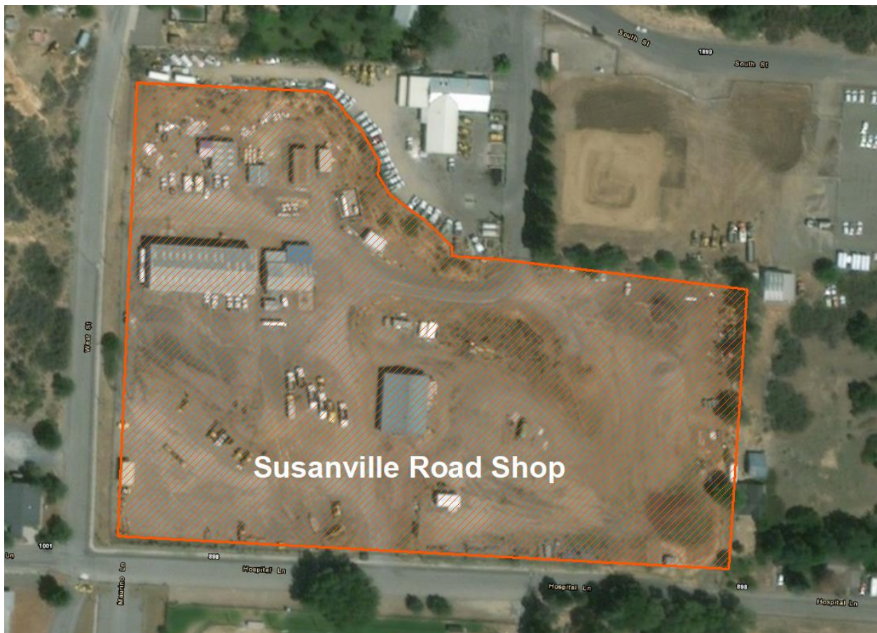
Figure 6.6 Susanville Road Shop
