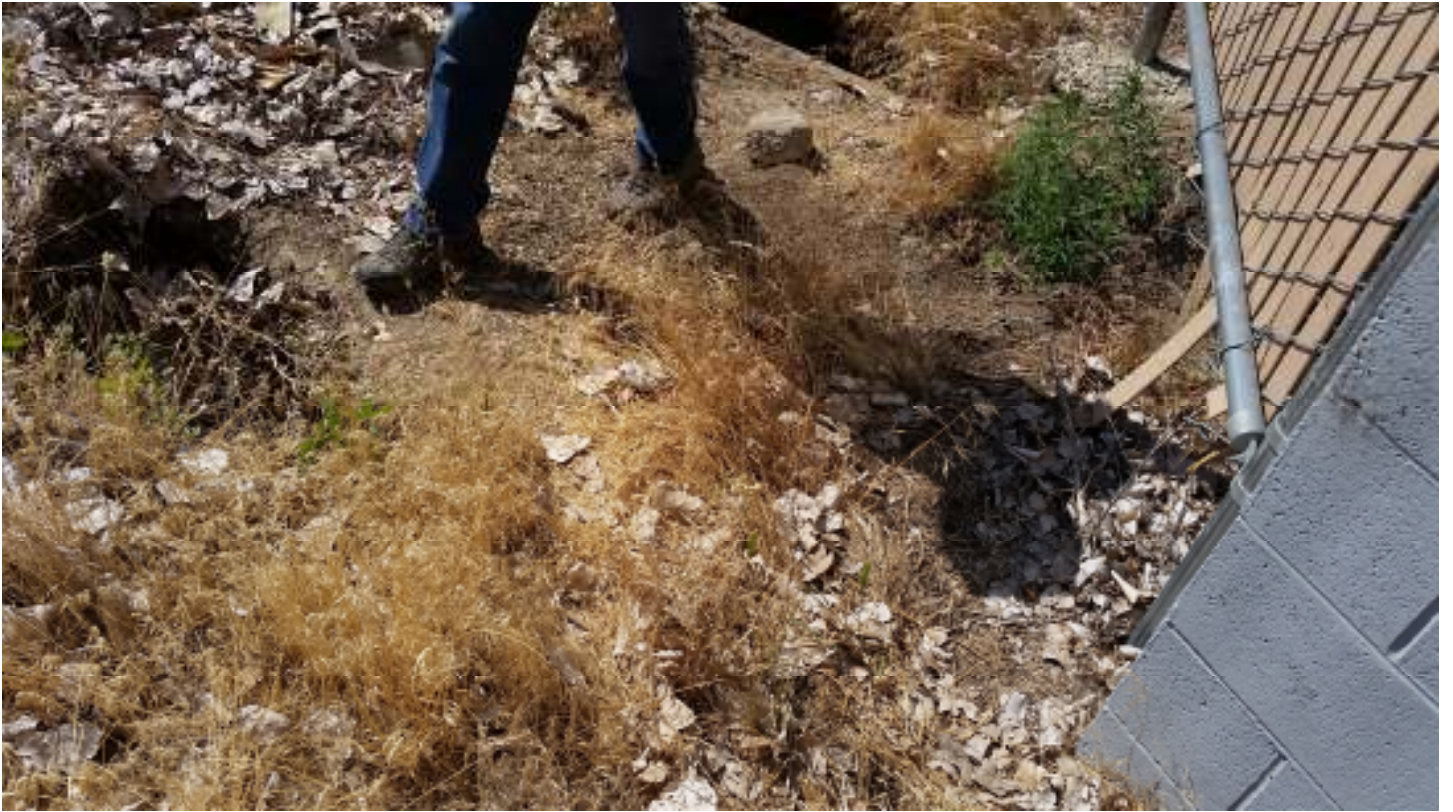
Figure 6 Drain Inlet to Drainage Ditch
