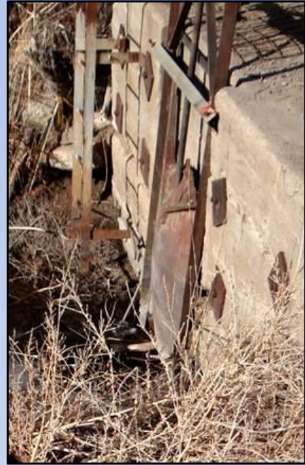
Old Channel headgate
