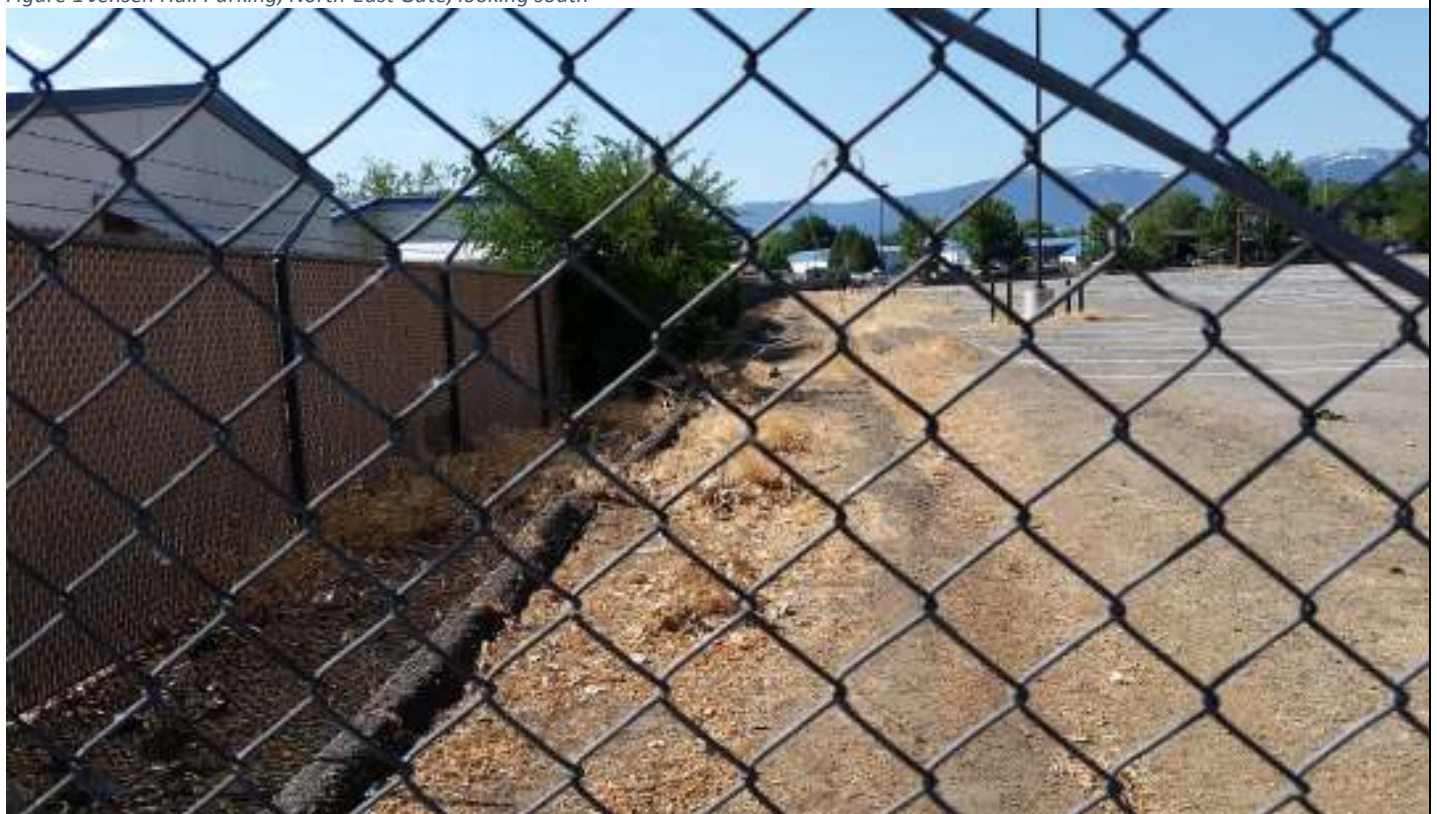
Figure 2 Jensen Hall Parking, Eastern fence, Curb (note lack of drainage infrastructure adjacent to mobile home park).
