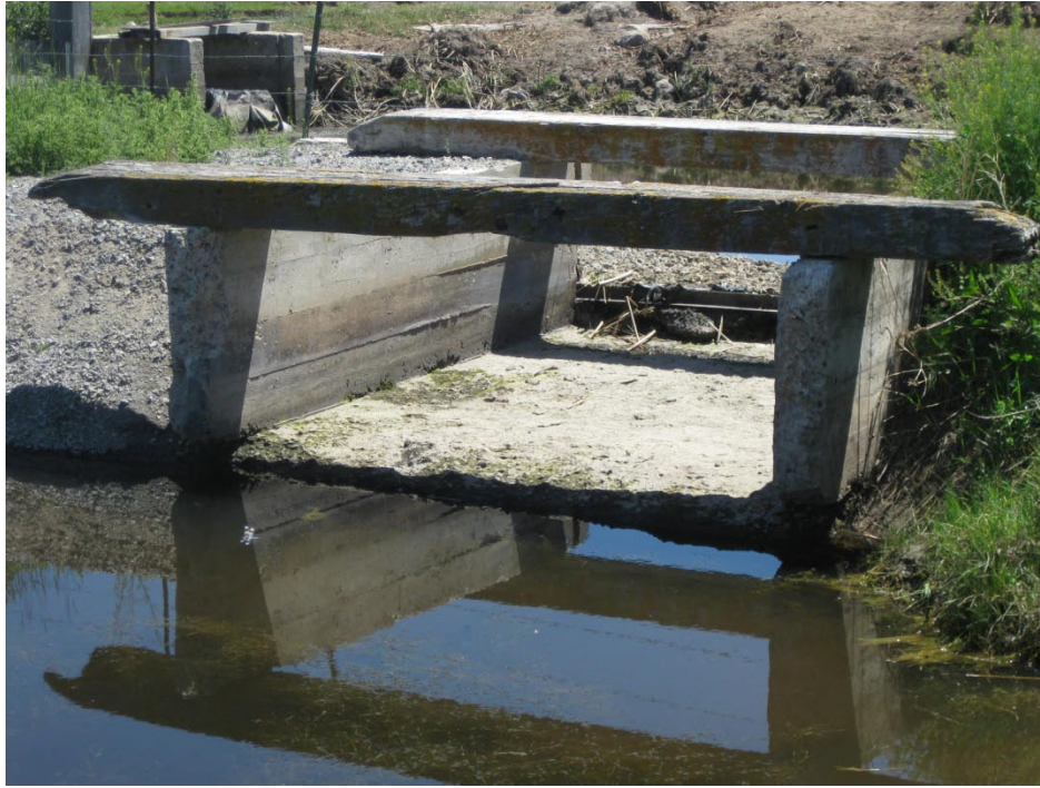
Figure 6: 100 Inch Weir on Willow Creek
