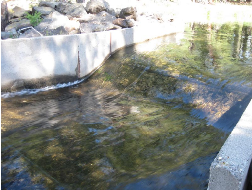
Figure 3: McCoy Flat Outlet 12' Parshall Flume
